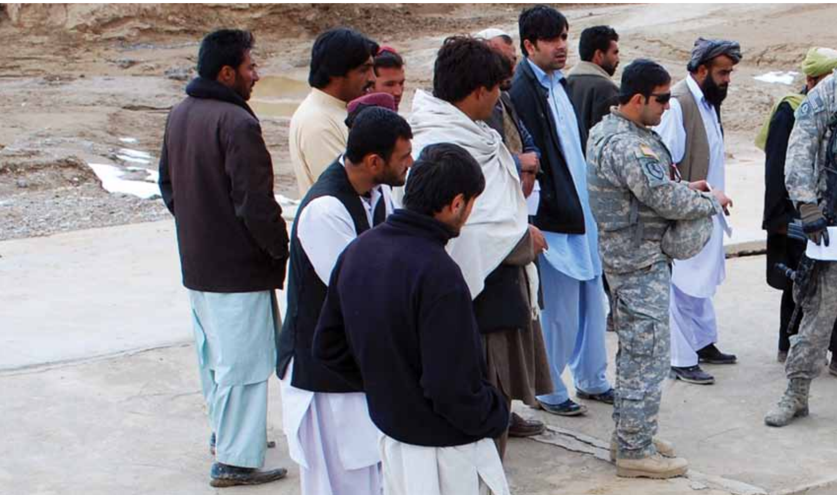
Provincial Reconstruction Team with contractors at bridge-repair job site, Zabol province, Afghanistan. (U.S. Air Force photo)
