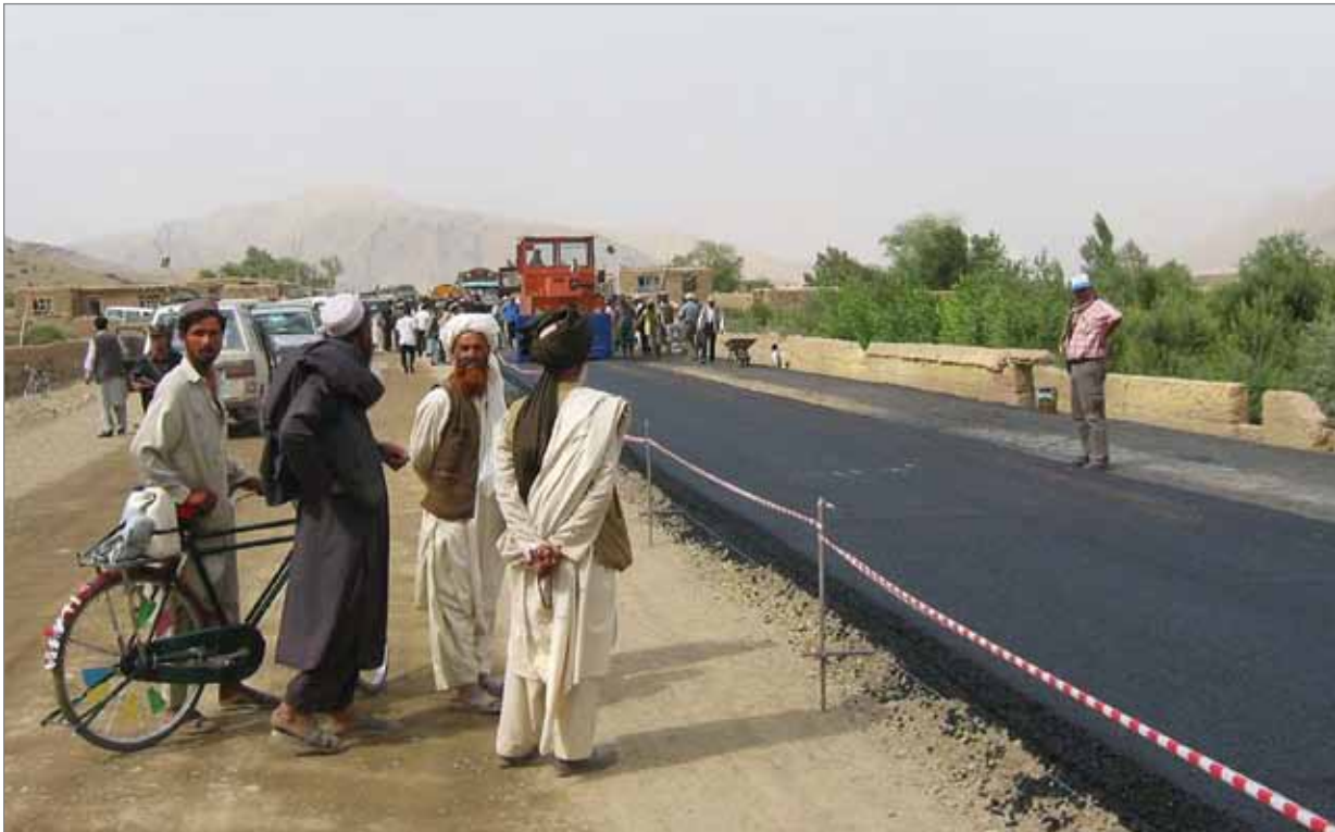
Kabul-to-Kandahar road construction, 2003. (USAID photo)
