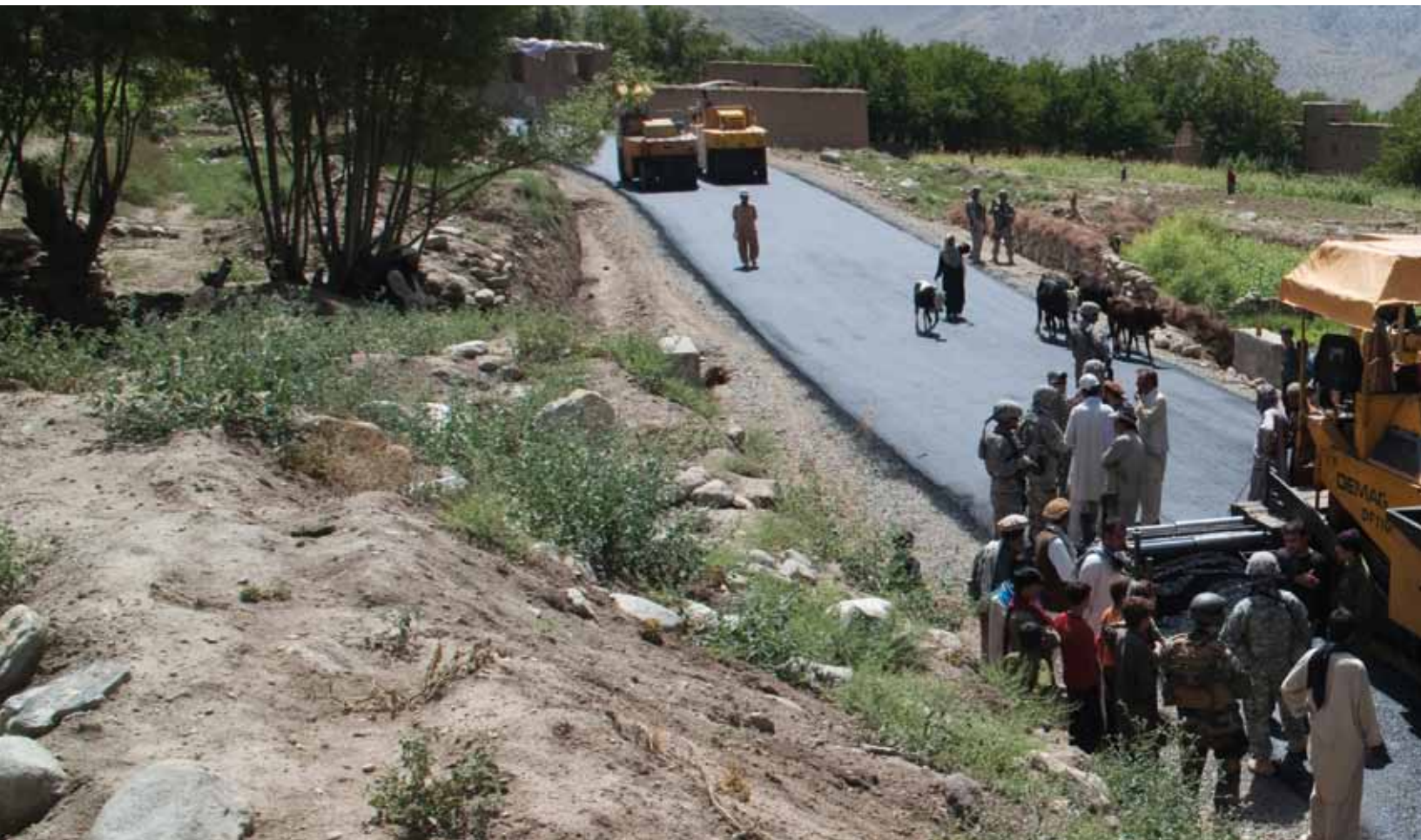
Road construction, Kapisa province, Afghanistan. (Defense photo)
